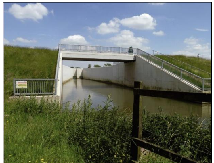
Flow control structure looking upstream towards the embankment
