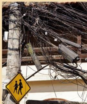
E Illegal electricity connections in a favela
